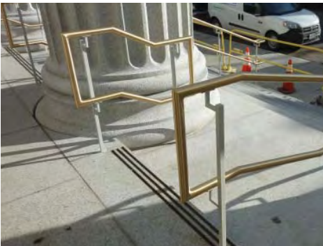
New top step scribed around the column
