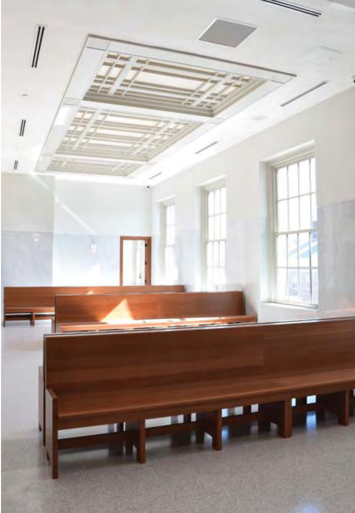
The original laylight was restored and relocated to the east wing waiting area.
