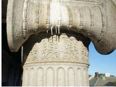
Existing condition - efflorescence
